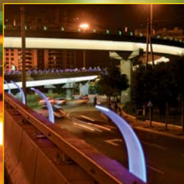
Olympic Parc, Beijing
