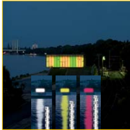
High-water Pumping Station, Cologne
